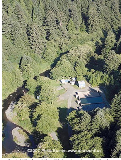
Aerial Photo of the Water Treatment Plant
