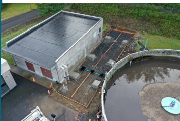
Foundation for the receiving container
